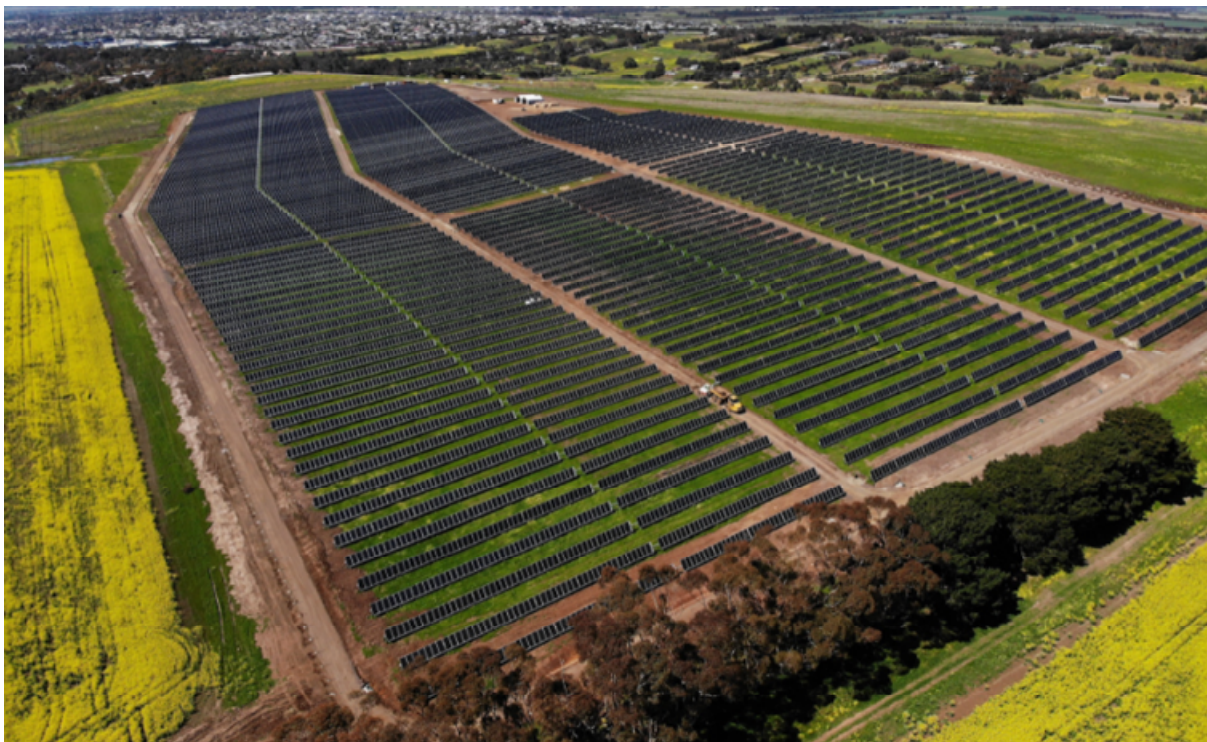
Figure 3: image showing under construction Solar Farm in Australia using Nextracker single axis tracking technology. Some slopes are up to 13 degrees, higher than slopes at the Proposal Site (Photo Courtesy of NGElectrical).
