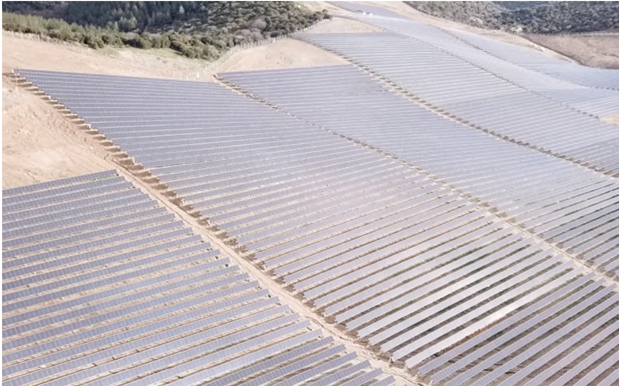
Figure 2: Image illustrating a newly constructed solar farm using Array Technology Trackers on slopes significantly greater than those found at the Proposal Site (up to 15 degrees North South and 35 degrees East/West, image courtesy of Array Technologies)
